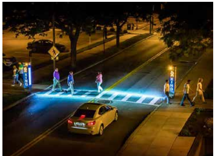
Image: LED-illuminated pedestrian crossing. (Source: Howard Industries)
